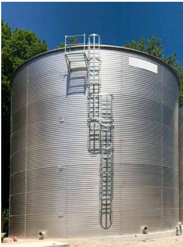
1.304 m 3 Bentonitsuspensionsspeicher in der Schweiz 1,304 m 3 Bentonite suspension tank in Switzerland
