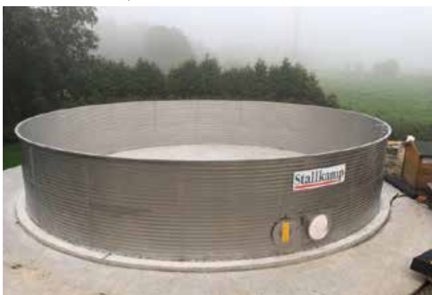
572 m 3 Klärschlammsspeicher aus Wellstahl 572 m 3 Waste water storage made from corrugated steel
