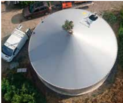
Membrandach von oben | Membrane roof from above
