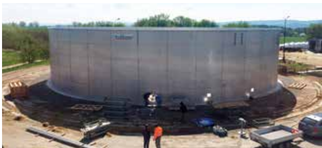
6.283 m 3 Wellstahlbehälter in Tschechien 6,283 m 3 Corrugated steel tank in the Czech Republic
