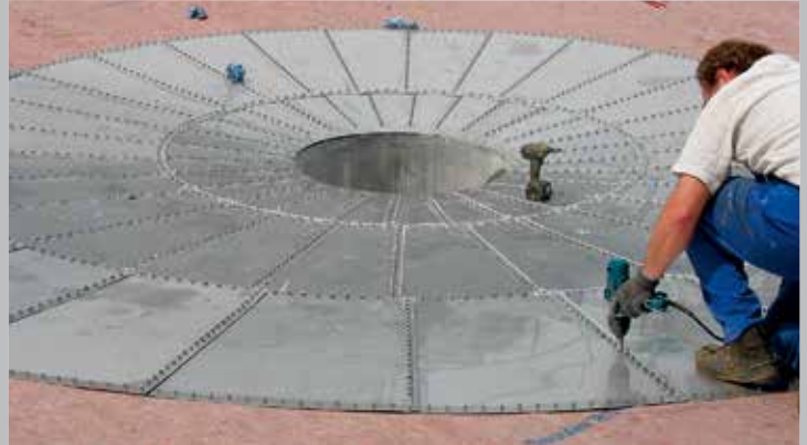
▶ Edelstahlboden in einem Abwasserbehälter ▶ Stainless Steel Bottom in a Wastewater Tank
